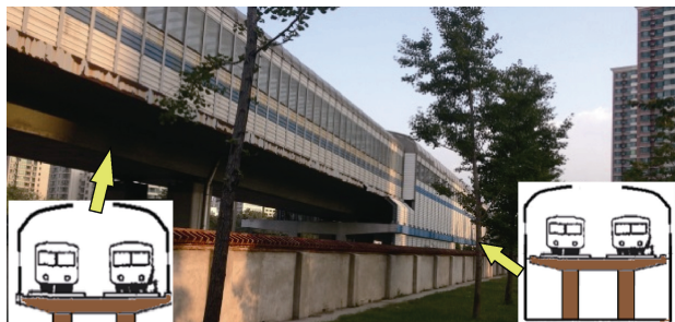
图3 北京地铁 13 号线某高架不同降噪措施段 Figure 3 Different noise reduction measures for a viaduct section of Beijing line 13
